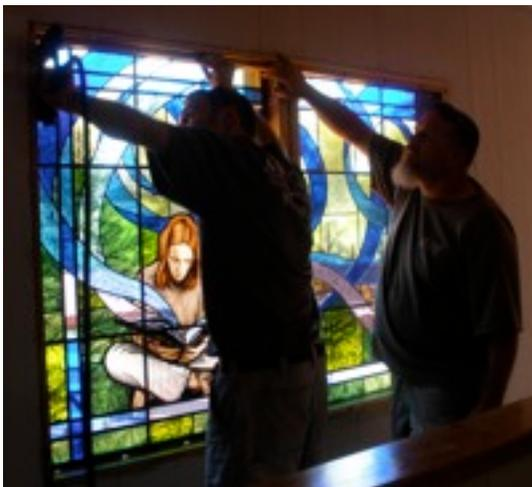
A&E Glass in Cresco helped with the install. Panes of tempered glass were installed on both sides of the stained glass for safety.
